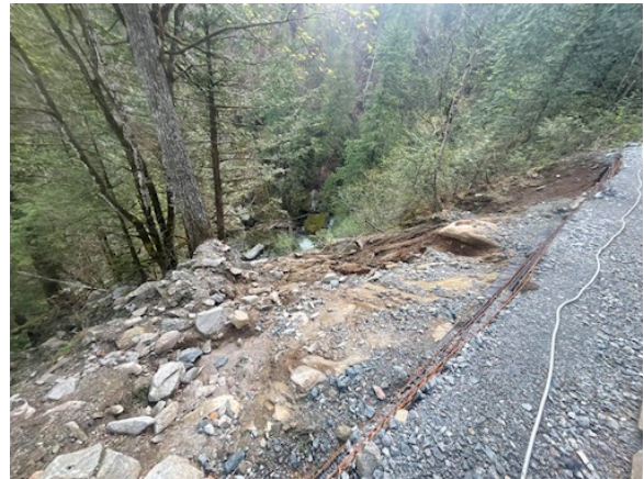
Slope below wall down to creek
